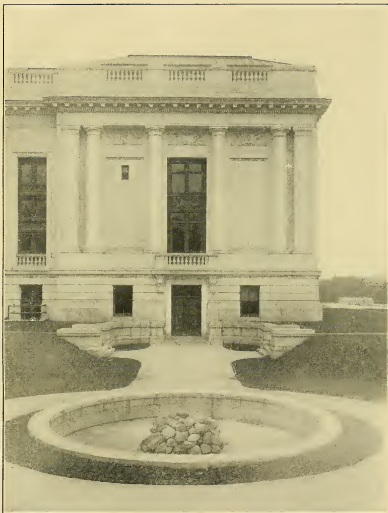
CONNECTICUT STATE LIBRARY AND SUPREME COURT BUILDING, HARTFORD. SECTION OF EAST FRONT.
